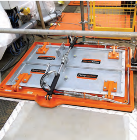
Hydraulic fire doors
