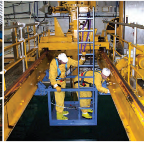
On-site OHTC work
