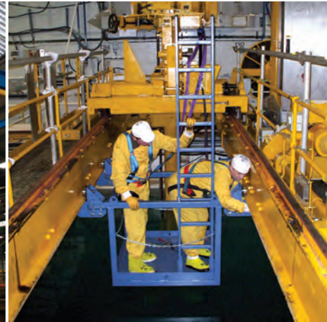
On-site OHTC work
